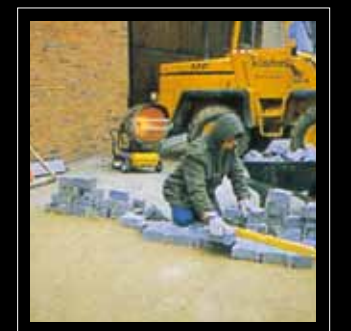
Winter construction: heats up materials, machines, and working sites
